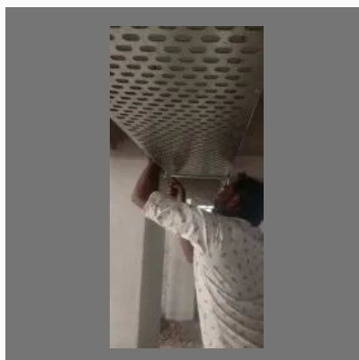
Installation Of Cable Tray
