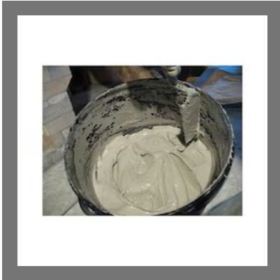
Mix Refractory Mortar
