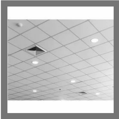
Grid False Ceiling Services
