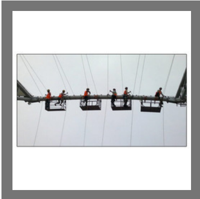
Membrane Installation Services
