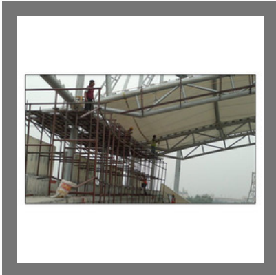
Membrane Installation Services
