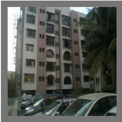
Building Structural Repair Service
