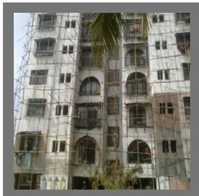
Industrial Wall Painting Service
