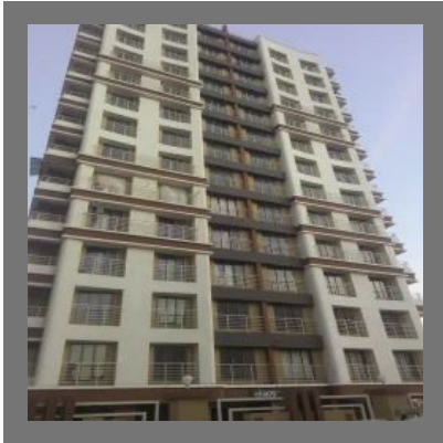
Building Painting Contractor Service
