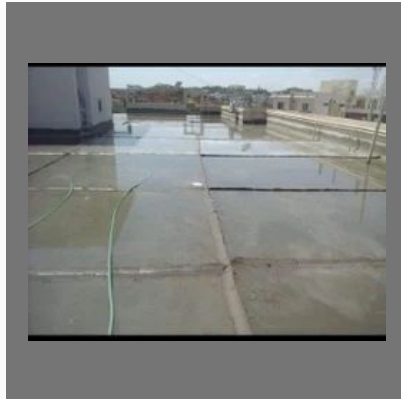
Terrace Waterproofing Service
