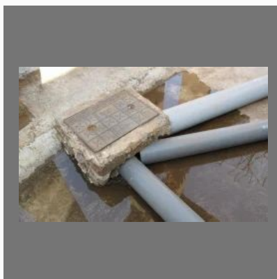
Building Plumbing Contractor Service
