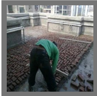
Water proofing services
