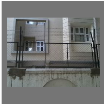
Wall Fencing With Chen Link net
