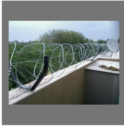
Concertina Wire Fencing Wall
