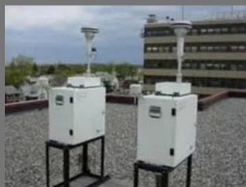
Infrastructure Engineering Services
