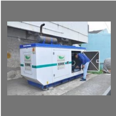
Kirloskar DG Repairing Service
