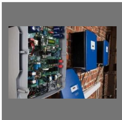
Elevator Inverter Repairing Service
