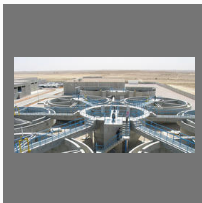
Waste Water Recycling Plants
