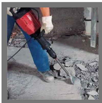
Concrete Chipping Service
