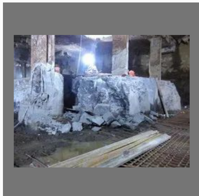
Rock Excavation with Blade/Wire Saw Cutting
