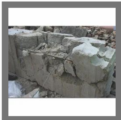
Concrete Demolition Service
