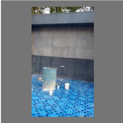
Wall Tile Installation Service
