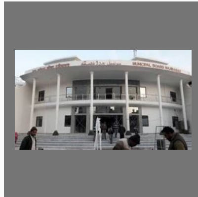
Aluminium Glazing Work
