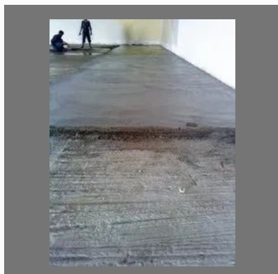
Floor Mortar Screed
