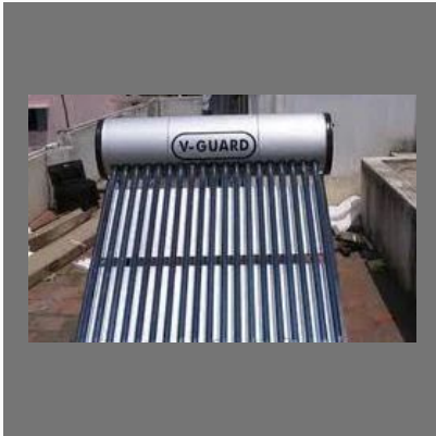
Solar Water Heater
