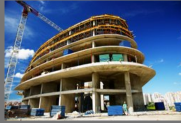
Hotel Building Construction Services
