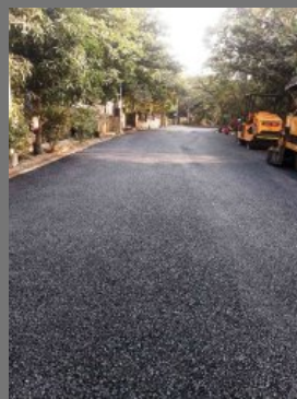
Dambar Road Construction Services
