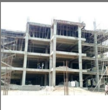
Hospital Building Construction Services
