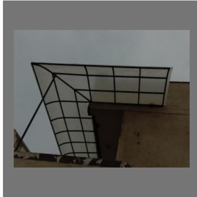
M S Fabrication Work
