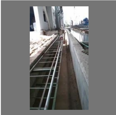
Stainless Steel Cable Tray Supply & Installation
