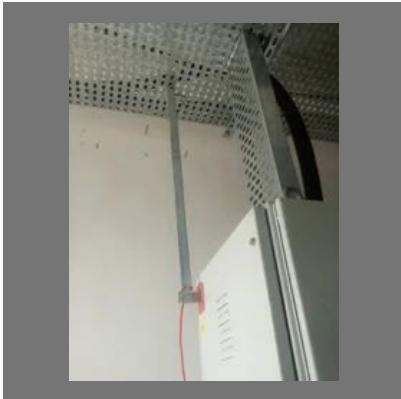
Supply And Installation Of Cable Tray And Wire
