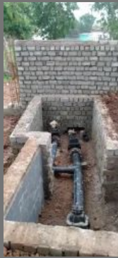
Overhead RCC Water Tanks Construction
