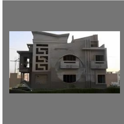
Hospital structure Building Construction
