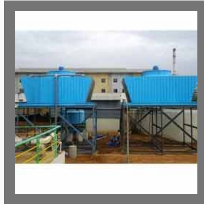
Pultruded FRP Cooling Tower
