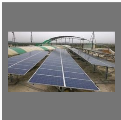
Solar Panel Mounting Structure Fabrication
