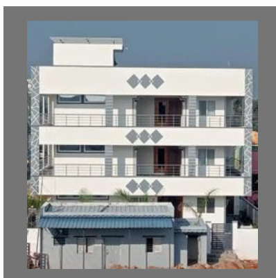
Commercial Construction Service
