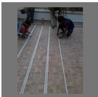
RCC Roof Waterproofing Treatment
