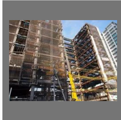
School Building Construction Service
