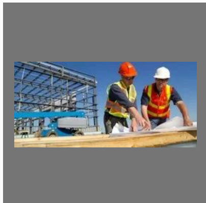
Industrial Civil Contractor Work
