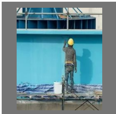
Exterior Wall Painting Service
