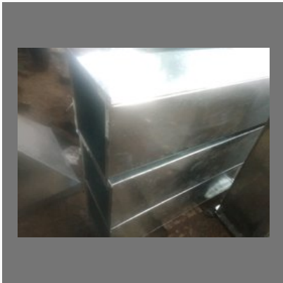
Gi Air Ducting
