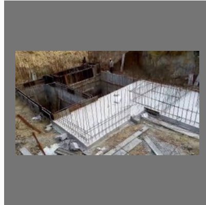
Sewage Treatment Plant Construction Service
