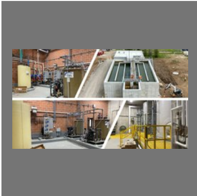
Water Treatment Plant Construction Service
