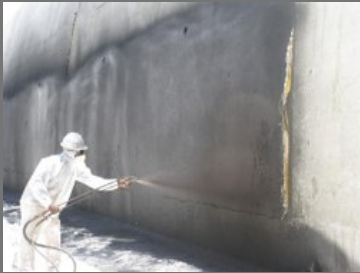
Commercial Waterproofing Service
