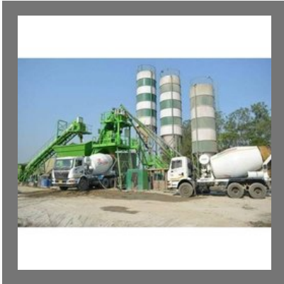
Construction Ready Mix Concrete
