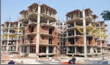
Apartment Construction Service
