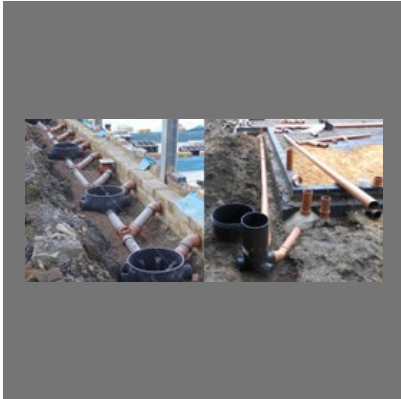
Drainage System Construction Service
