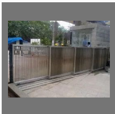
Telescopic Sliding Main Entrance Gate
