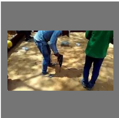
Anti Termite Treatment
