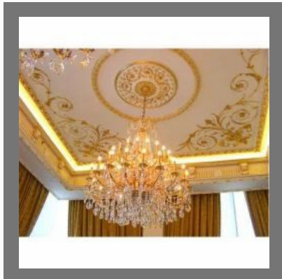
Decorative False Ceiling
