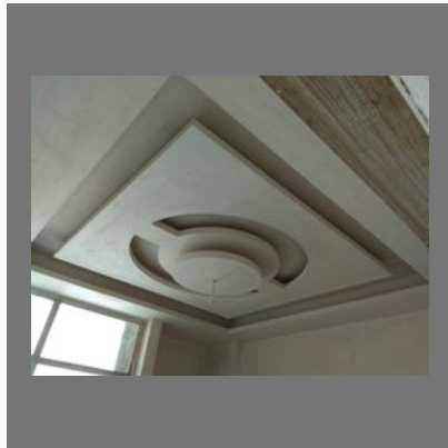
POP Fall Ceiling Work Services
