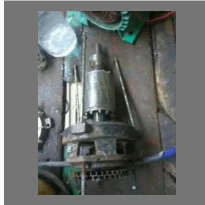
Water Motor Repairing
