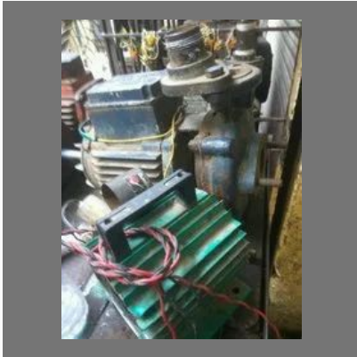
Water Pump Repairing
