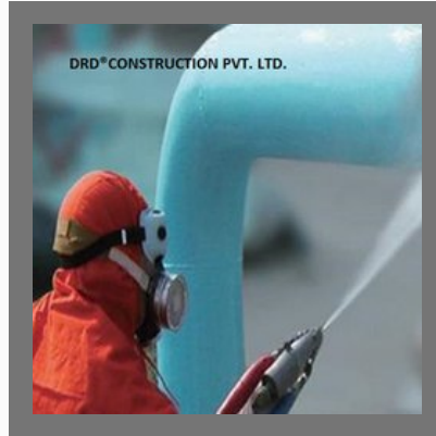
PU Coating On Structure
