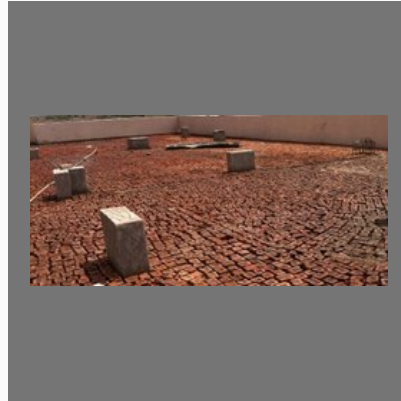
Brick Bat Waterproofing
