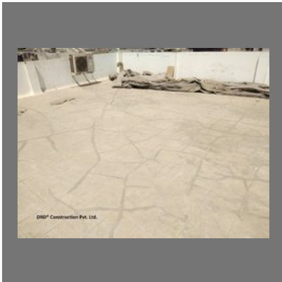
Crack Filling Service
