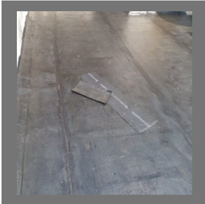
APP Membrane Waterproofing
