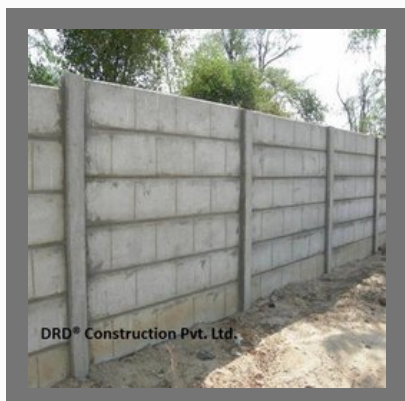
Compound Wall Services
