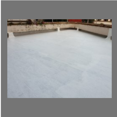
Terrace Cool Coating Services
