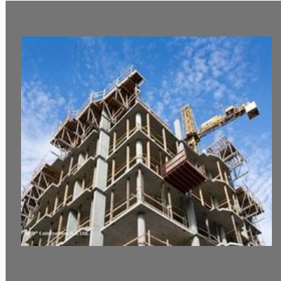
Civil Construction Contractor
