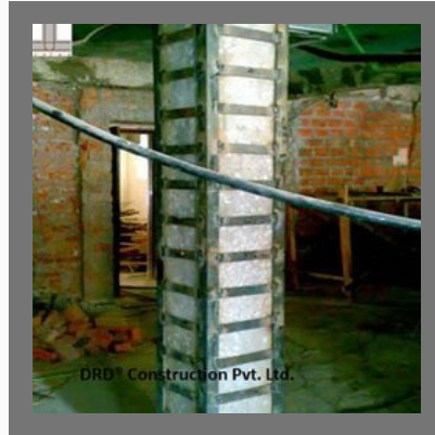
Structure Strengthening Work
