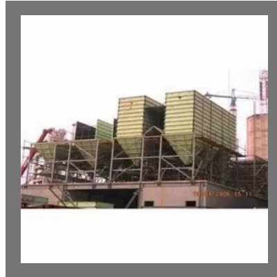
Cement Clinker Cooler Baghouse Filter
