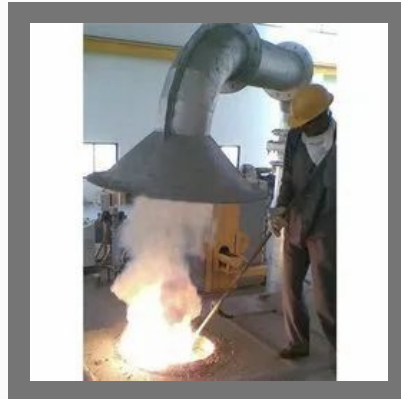
Fume Extraction System
