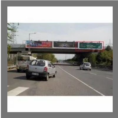
Flyover Panel Hoarding
