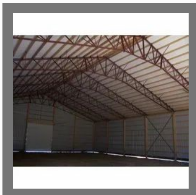
Steel Factory Sheds
