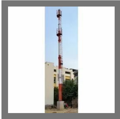
Monopole Communication Tower
