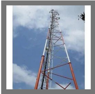
Three Legged Tubular Tower
