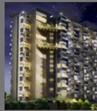
3 BHK Apartment Construction Services
