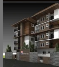
2 BHK Apartment Construction Services
