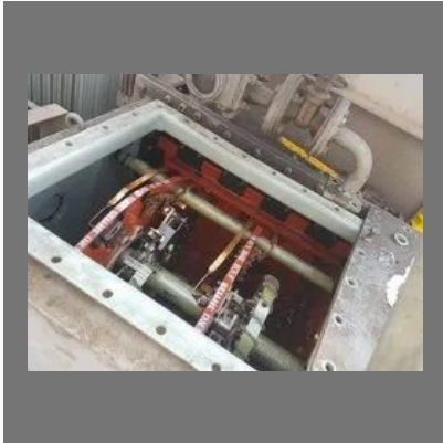
OLTC Overhauling Repairing
