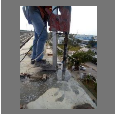
Diamond Slab Cutting Services
