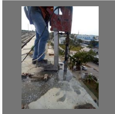
RCC Core Cutting Service
