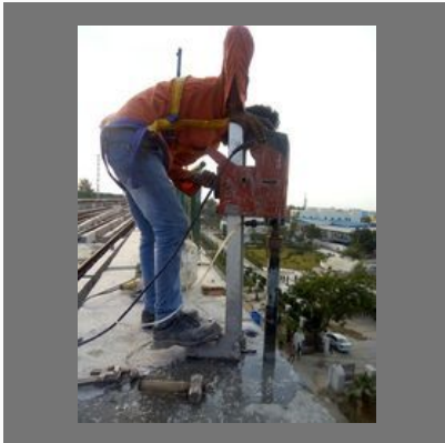
Diamond Core Cutting Works
