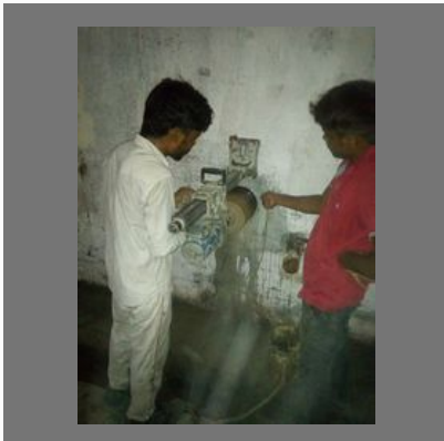
Concrete Core Drilling Services
