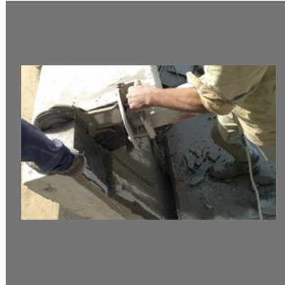
Concrete Core Cutting Services
