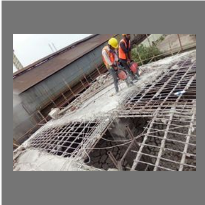
Concrete Slab Cutting Service
