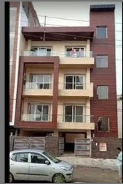
Aluminium Composite Panel Cladding Service
