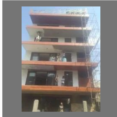
HPL Building Wall Cladding Service
