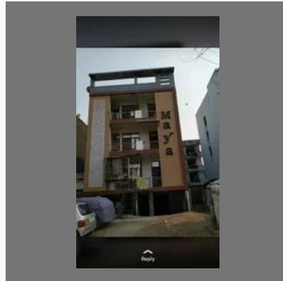
HPL Building Wall Cladding Service
