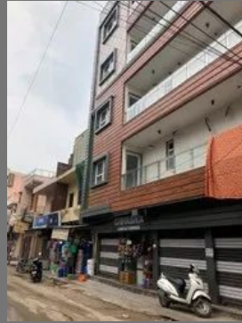
Aluminium Composite Panel Cladding Service
