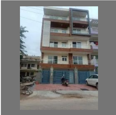
HPL Building Wall Cladding Service
