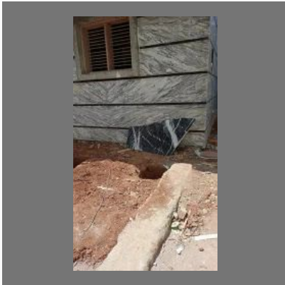
Italian marble onex fixing laying contact
