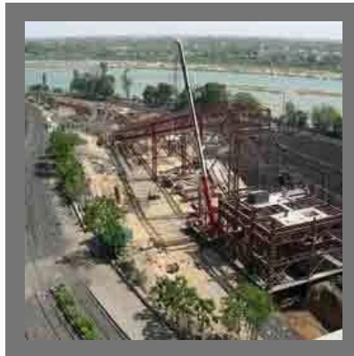
100 MT. Tyre Mounted Telescopic Boom Crane
