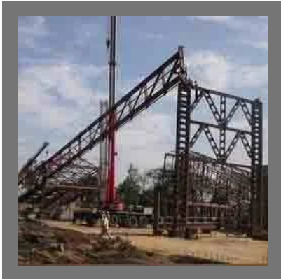
Mounted Telescopic Boom Crane
