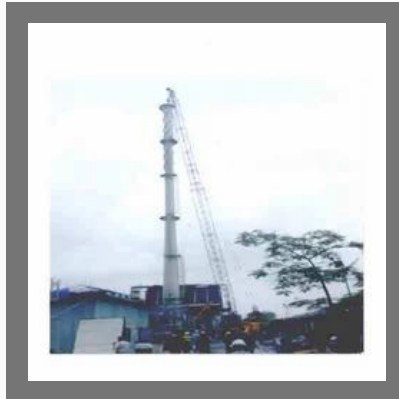
150 Mt. Crane Erecting Chimney Height : 72 Meter Main Boom
