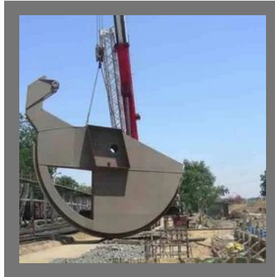
100 MT Tyre Mounted Telescopic Boom Crane Handling
