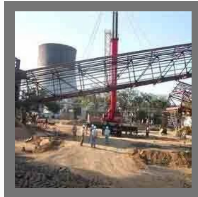
Mounted Telescopic Boom Crane
