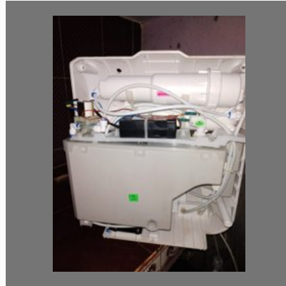
RO Purifier Repair Service
