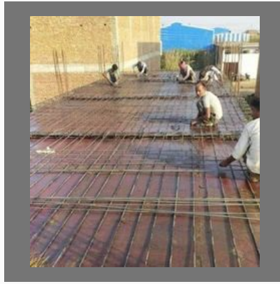
Warehouse Buildings Construction Services
