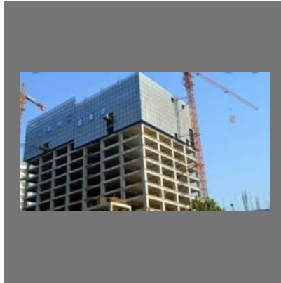
Hotel Construction Work
