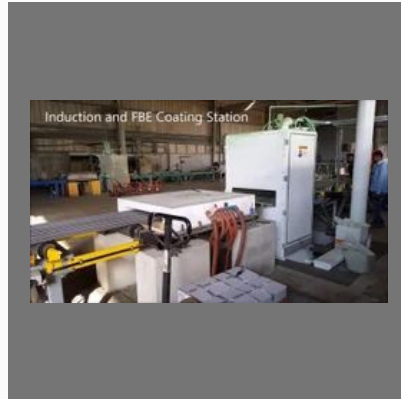
Rebar Coating Plant
