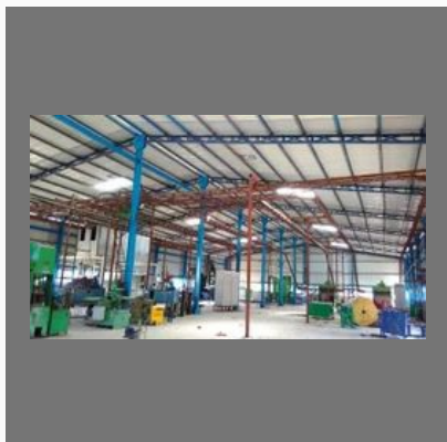
Industrial Steel Shed
