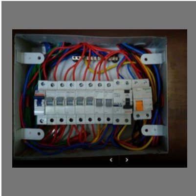
Electric Wiring Installation Service For Corporate Office
