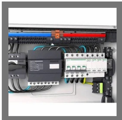
Electric Surge Protection Device Installation Service
