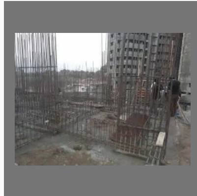
IPS And RCC Work Services
