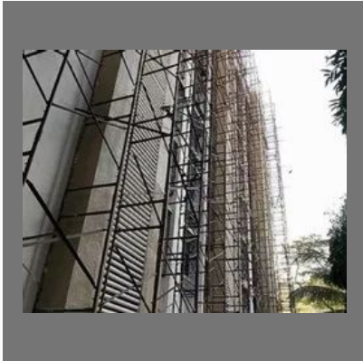
Building Structural Repair Services
