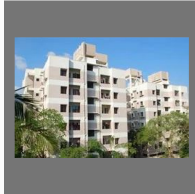
F Type Quarters Construction Service
