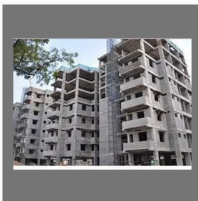
Construction Of F Type Quarters
