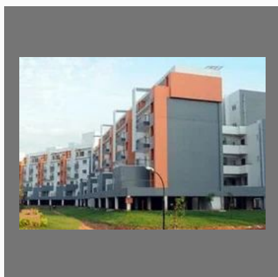
Commercial Building Construction Service
