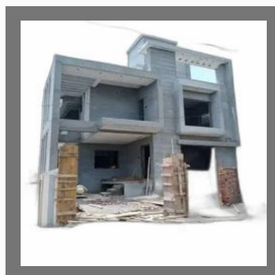
Residential Construction Service
