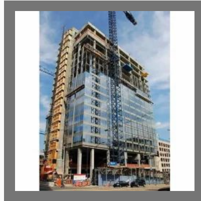
Hotel Construction Service
