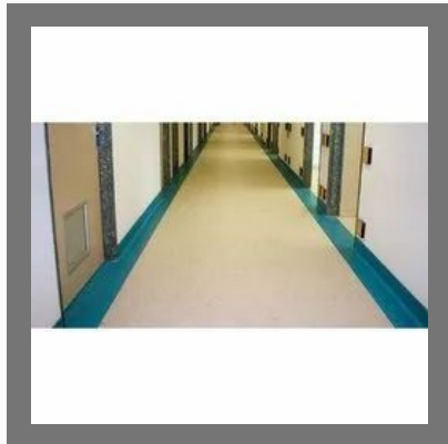
Operation Theatre Flooring
