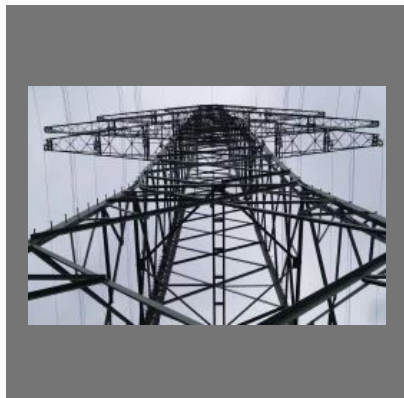
Electrical Turnkey Solution
