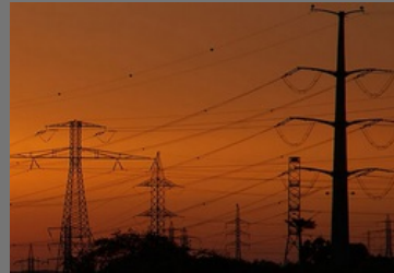
Co- Power Generation
