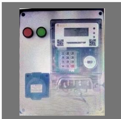
Electric Vehicle Ev Charging Station
