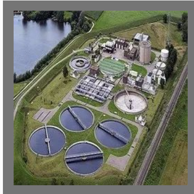
Common Effluent Treatment Plant ( CETP)
