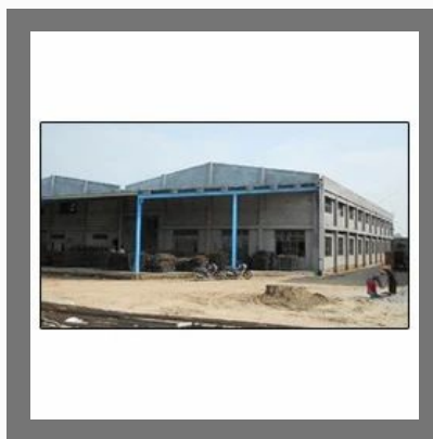
Tyres Plant Construction Service
